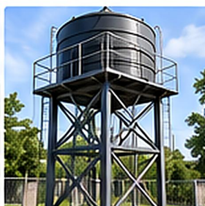
Overhead Tank Structures
