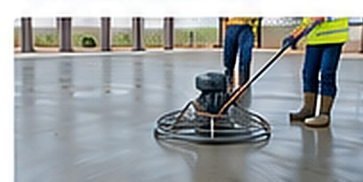
Industrial Flooring / PQC
